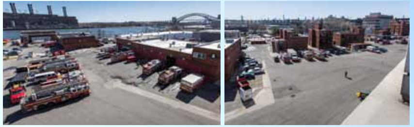
FDNY Fire Academy is located on Randalls Island
